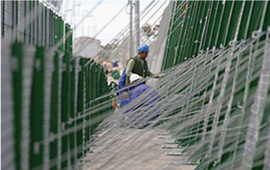
Figure 6.5: Steel cable system in Melilla
